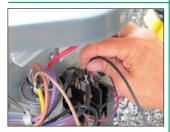
9] Attach the flagged end of the black wire to the Compressor Common on the "T" side of the contactor.
