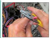
4] Strip the compressor Run wire at least 1/2 in.\* Crimp appropriate size Ferrule (supplied) onto it.
