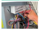
13] Remove the loose wire (from Step 7) from the active input of the contactor and attach the stripped end of the Active wire in its place.
