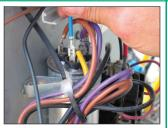
11] Attach the flagged end of the blue wire to the other terminal#2 of the Run Capacitor. Ensure that this terminal on the capacitor also joins to the Start Winding of the compressor.
